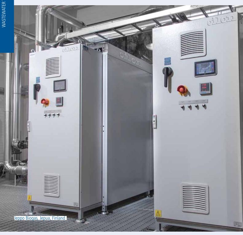
"Energy efficiency of the biogas plant has been improved with Oilon's industrial ChillHeat pumps and direct heat recovery. The process is cooled and heated with the heat pumps to minimize the need to use primary energy."
