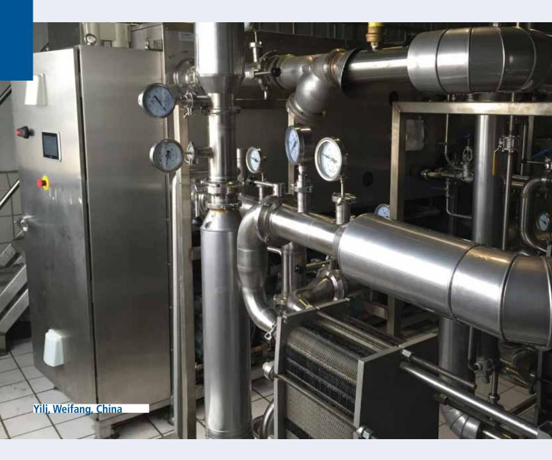
"At the factory of China's largest dairy company Yili in Weifang, a heat pump has been integrated into the precooling and preheating system to improve energy efficiency."
