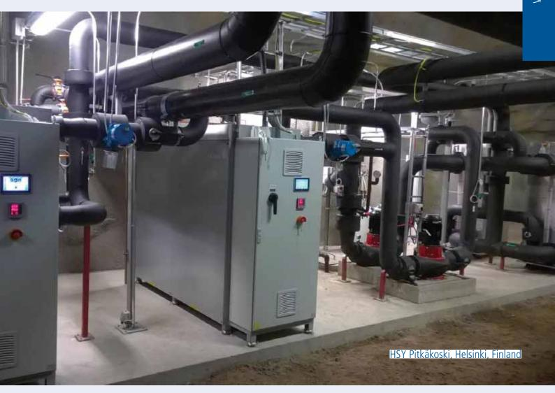
"The waste heat from the wastewater is used to heat the treatment plant facility with industrial ChillHeat pumps."
